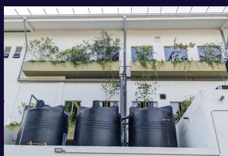
Rainwater harvesting facility
